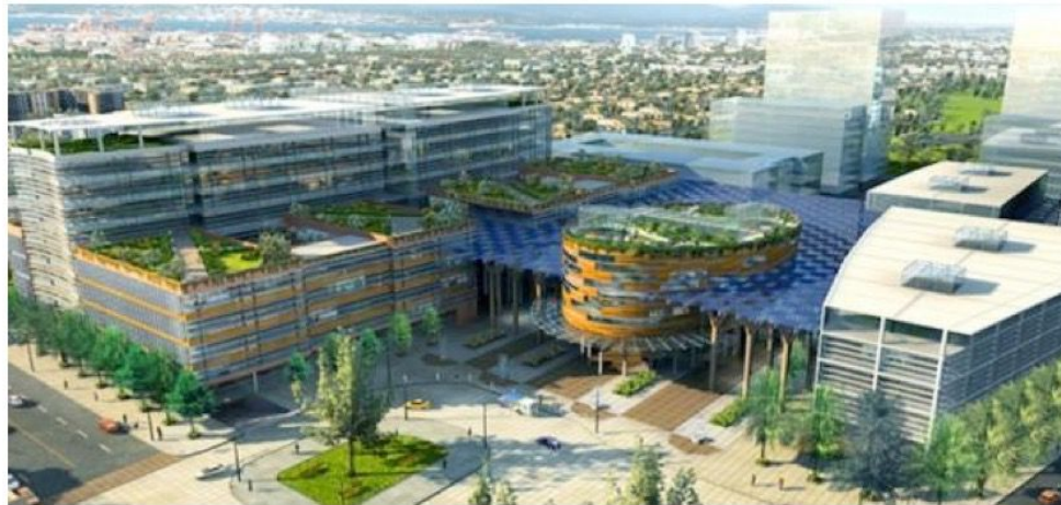
New Construction of St. Paul's Hospital.
